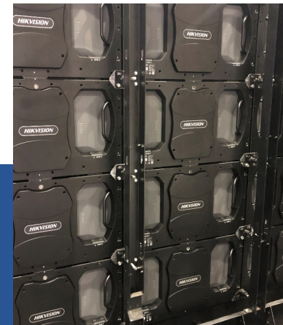
Improving the aesthetics of the installation on the site, and eliminating potential safety hazards caused by excessive wiring
